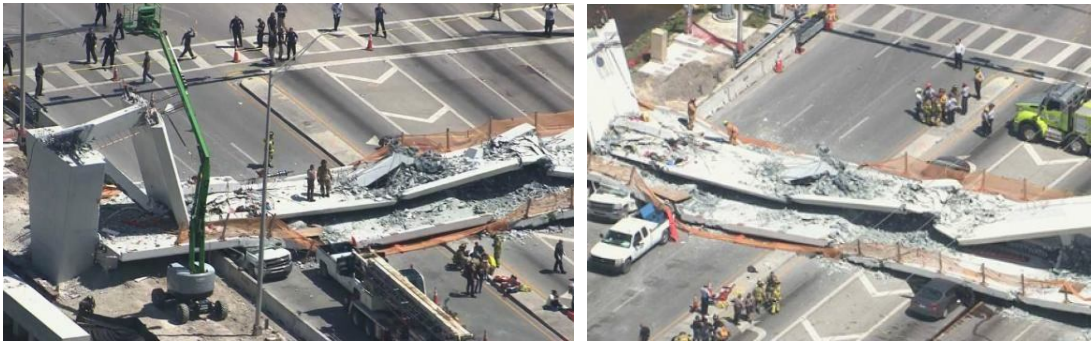
Fig. 1. Pedestrian bridge collapse in Miami, Florida. 2018
