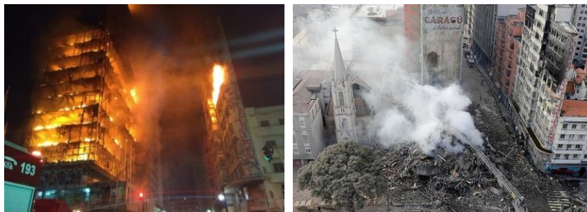
Fig. 1. Multi-storey building collapse due to a fire in Sao Paulo, Brazil, 2018
